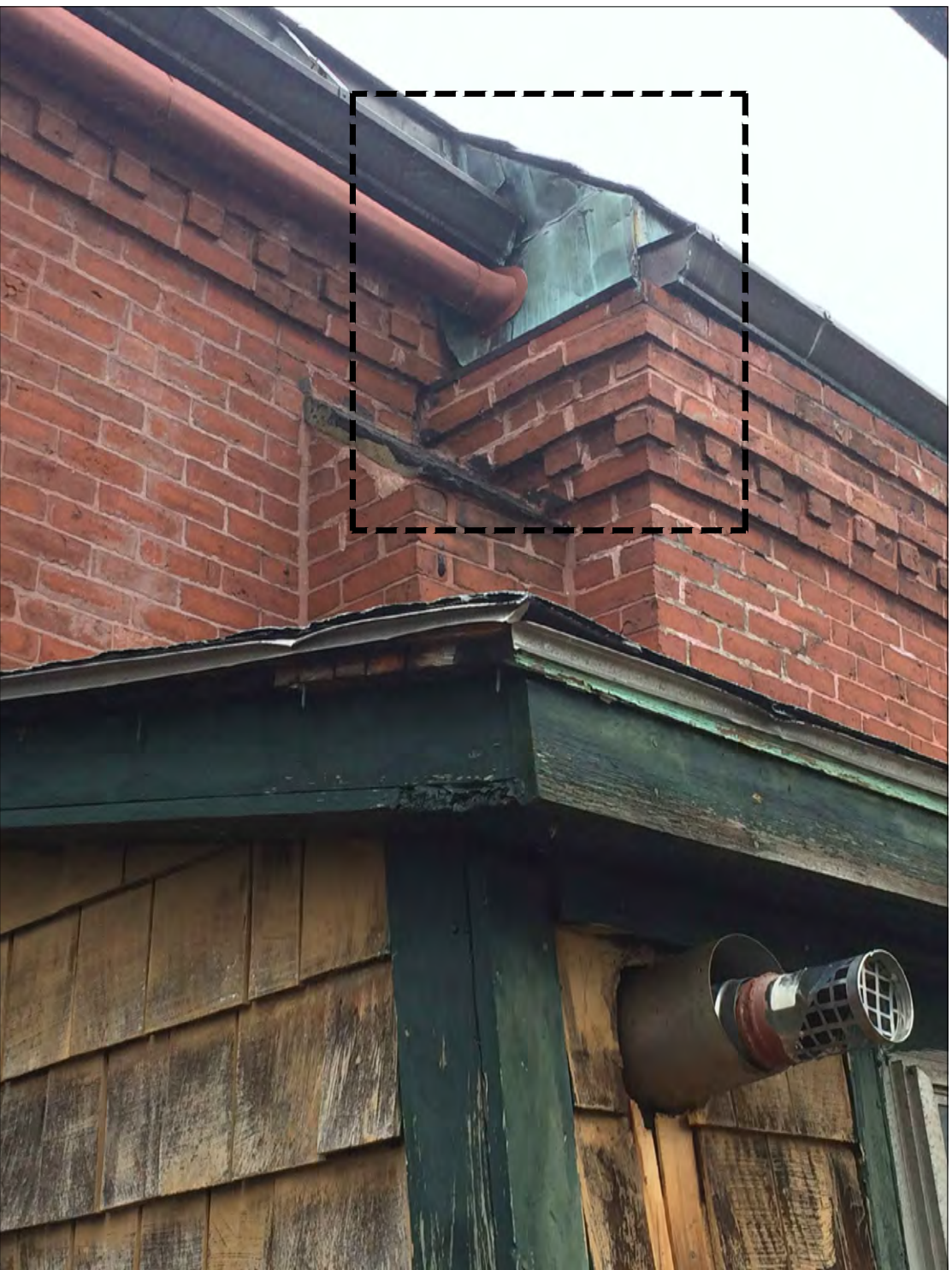
PHOTO 4/DRAWING D-200: Note different gutter and corbel heights at south elevation above bulkhead.
