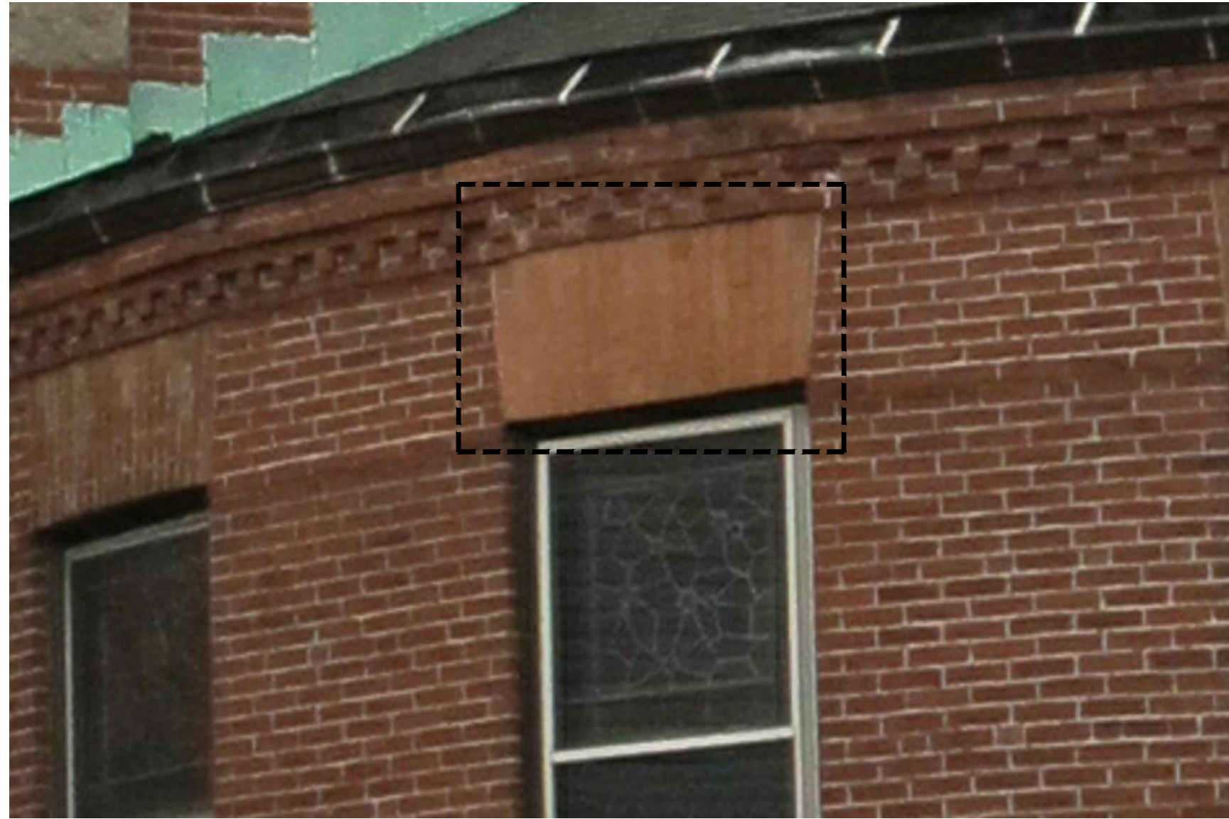
2 MISMATCHED BRICK AT FLAT ARCH - SOUTH ELEVATION (AREA INDICATED)
