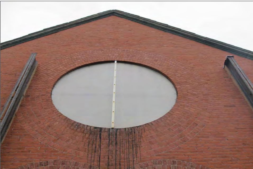
PHOTO 6/DRAWING D-200: Asphalt sealant stained masonry below circular window.
