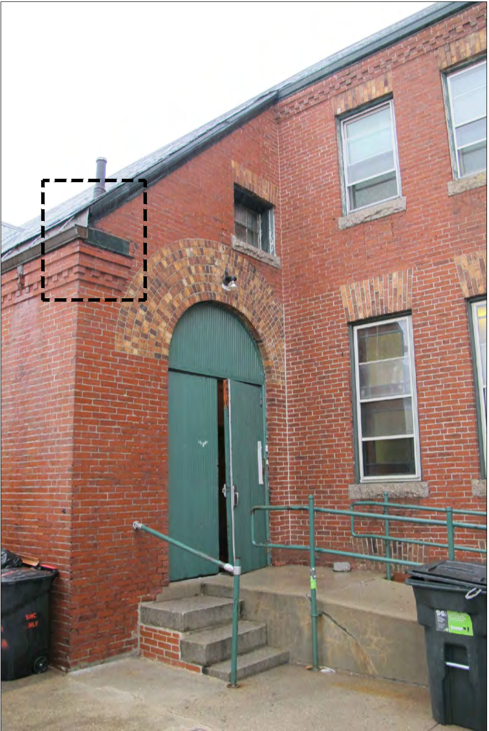
PHOTO 9/DRAWING D-201: Missing roof rake return at southeast elevation.
