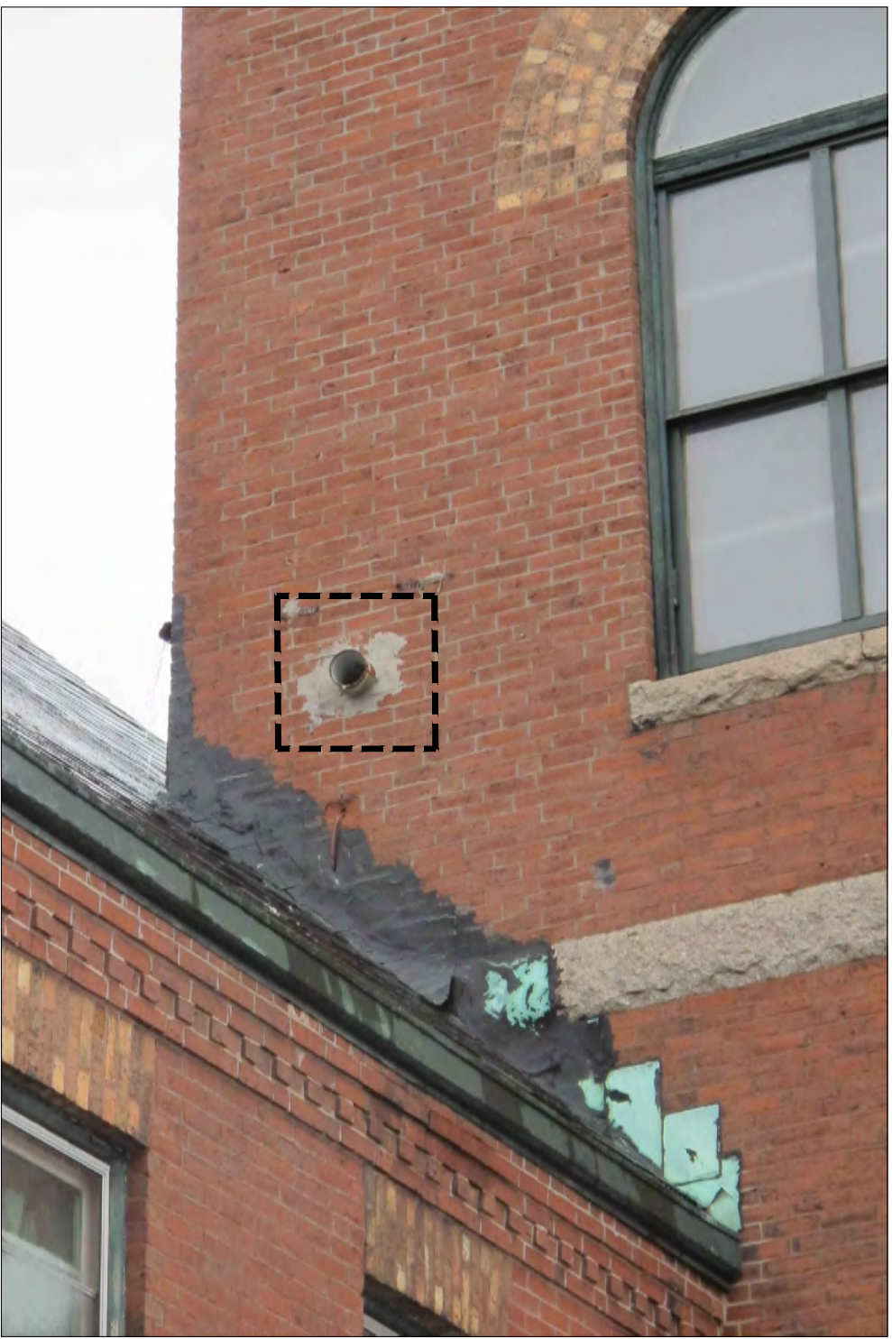
PHOTO 2/DRAWING D-201: Damaged masonry and projecting roof drain at northeast elevation.
