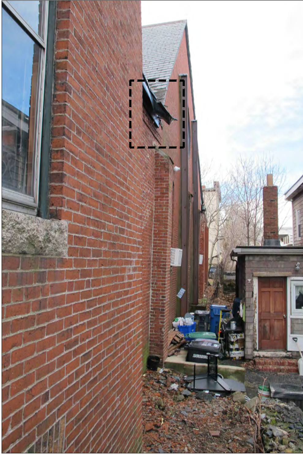
PHOTO 1/DRAWING D-200: Damaged flashing and gutter adjacent to cross-gable at the north elevation.
