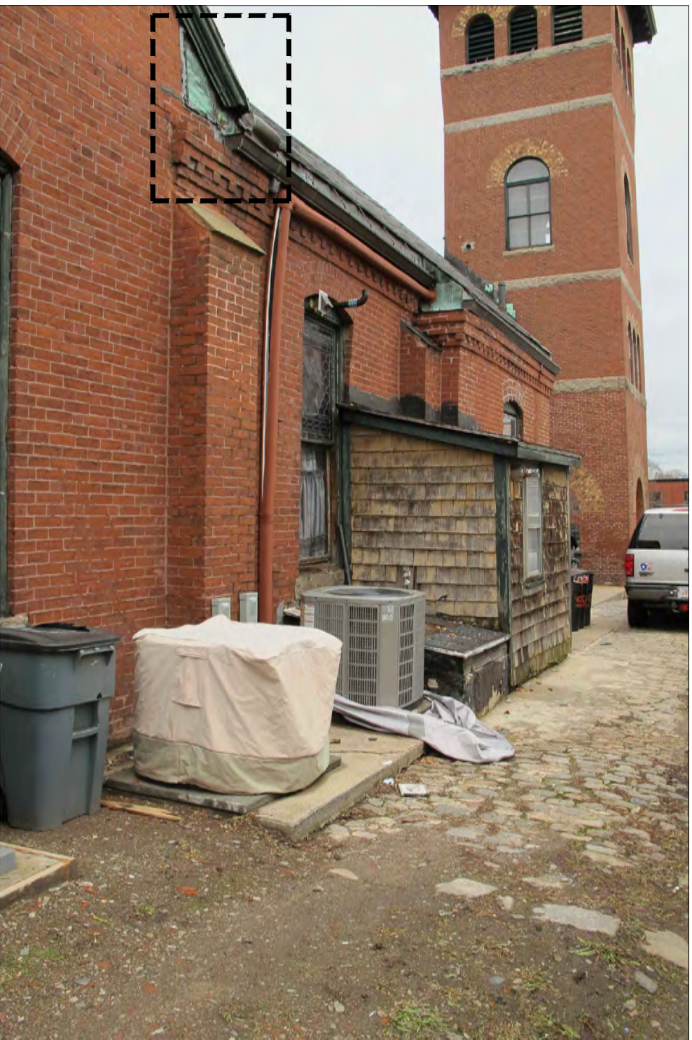
PHOTO 3/DRAWING D-200: Missing roof rake return and gutter.
