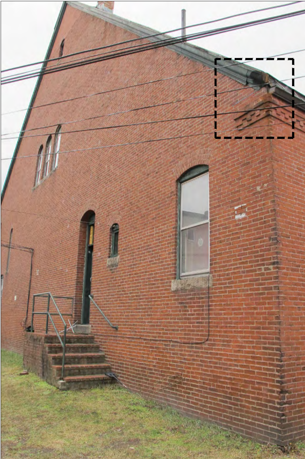
PHOTO 8/DRAWING D-201: Missing roof rake return at west elevation, (right hand side).
