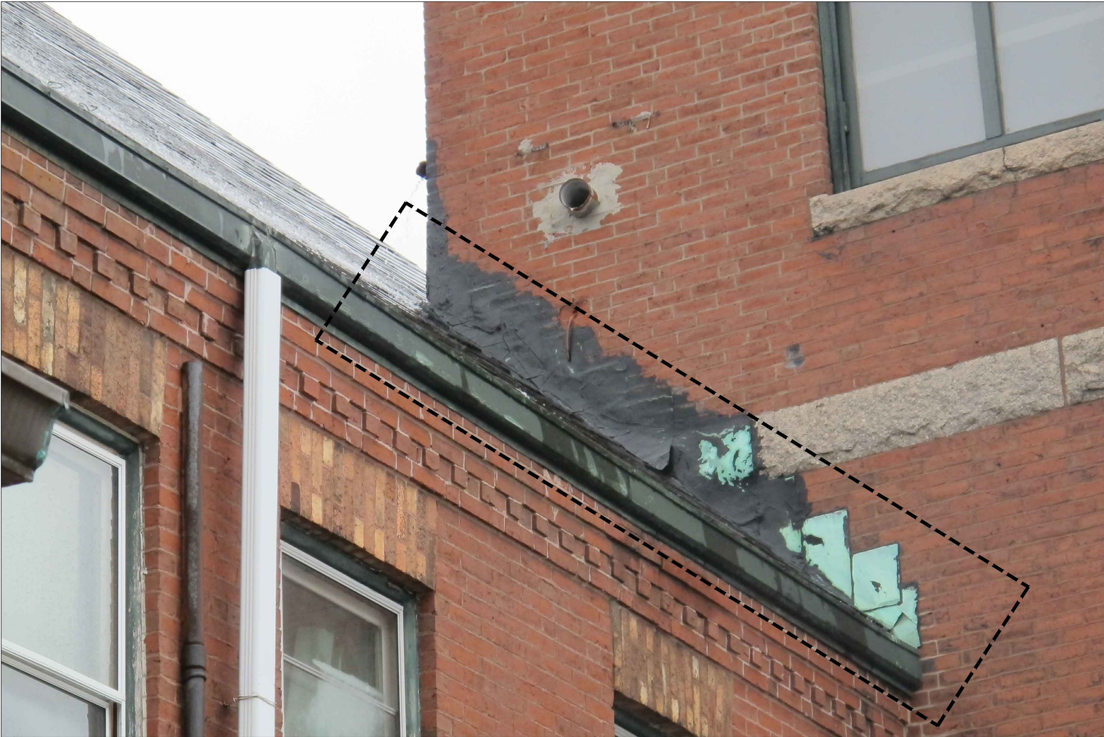
PHOTO 10/DRAWING D-201: Asphalt roofing sealer and step flashing at northeast elevation.
