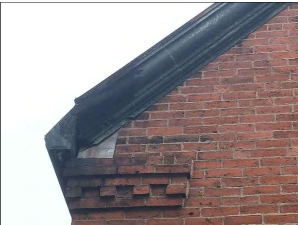
PHOTO 5/DRAWING D-201: Missing roof rake return at west elevation, (left hand side).
