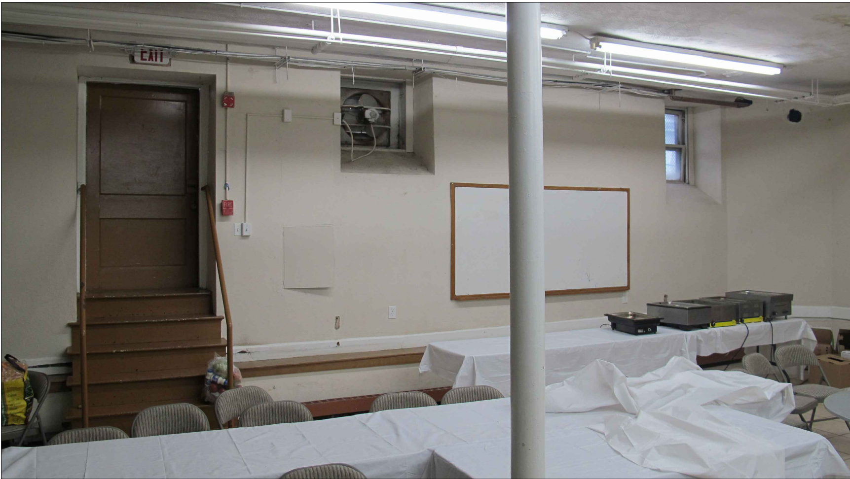
PHOTO 3: Existing Social / Dining area at basement. The existing floor elevation will be raised to match adjacent Kitchen and Stage floor elevations.
